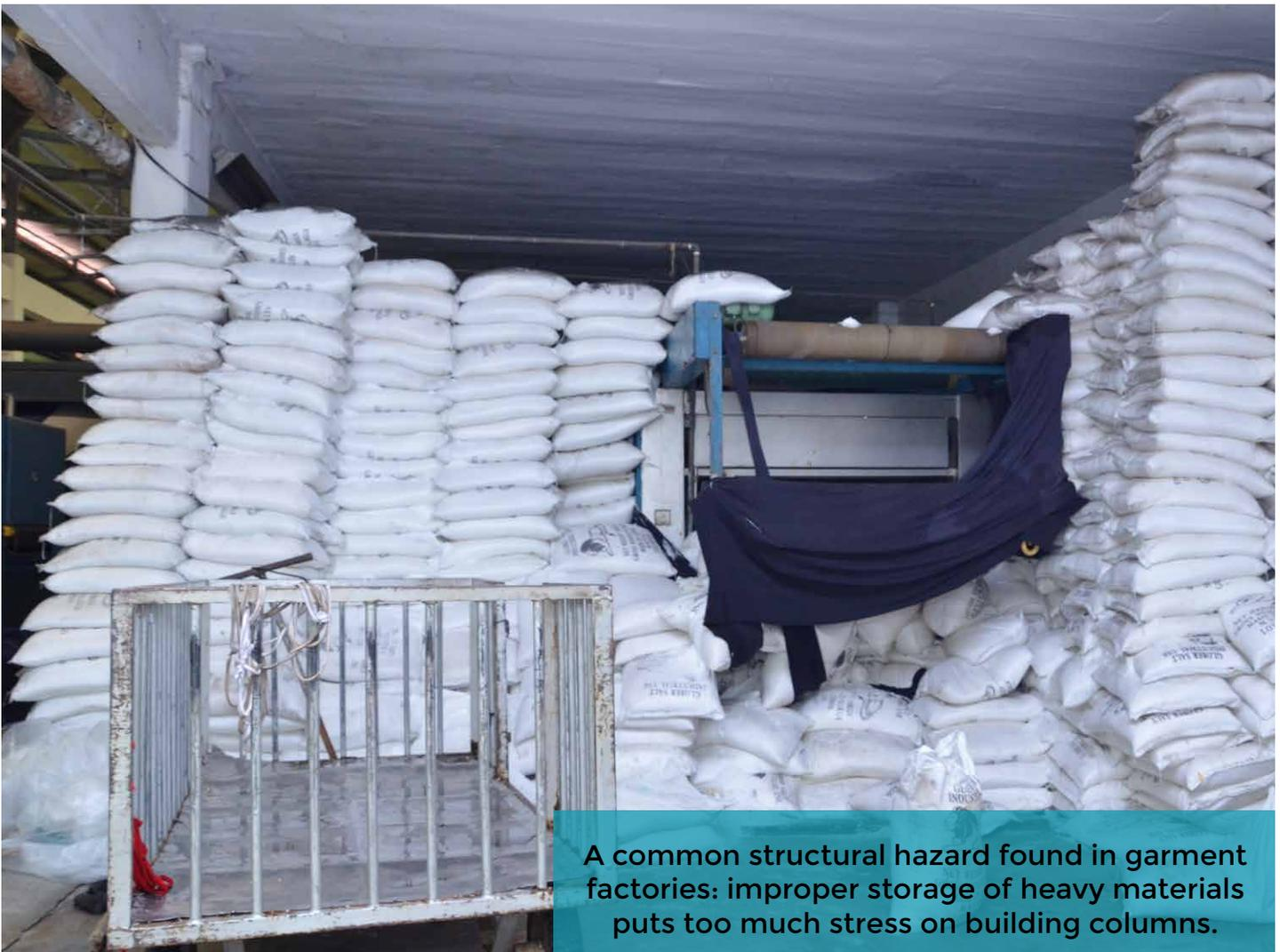
A common structural hazard found in garment factories: improper storage of heavy materials puts too much stress on building columns.
